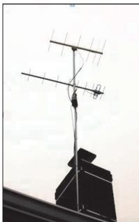
The smaller antennas, 1.25m and 70cm, were put on a rotator and strapped to the chimney. This was the
